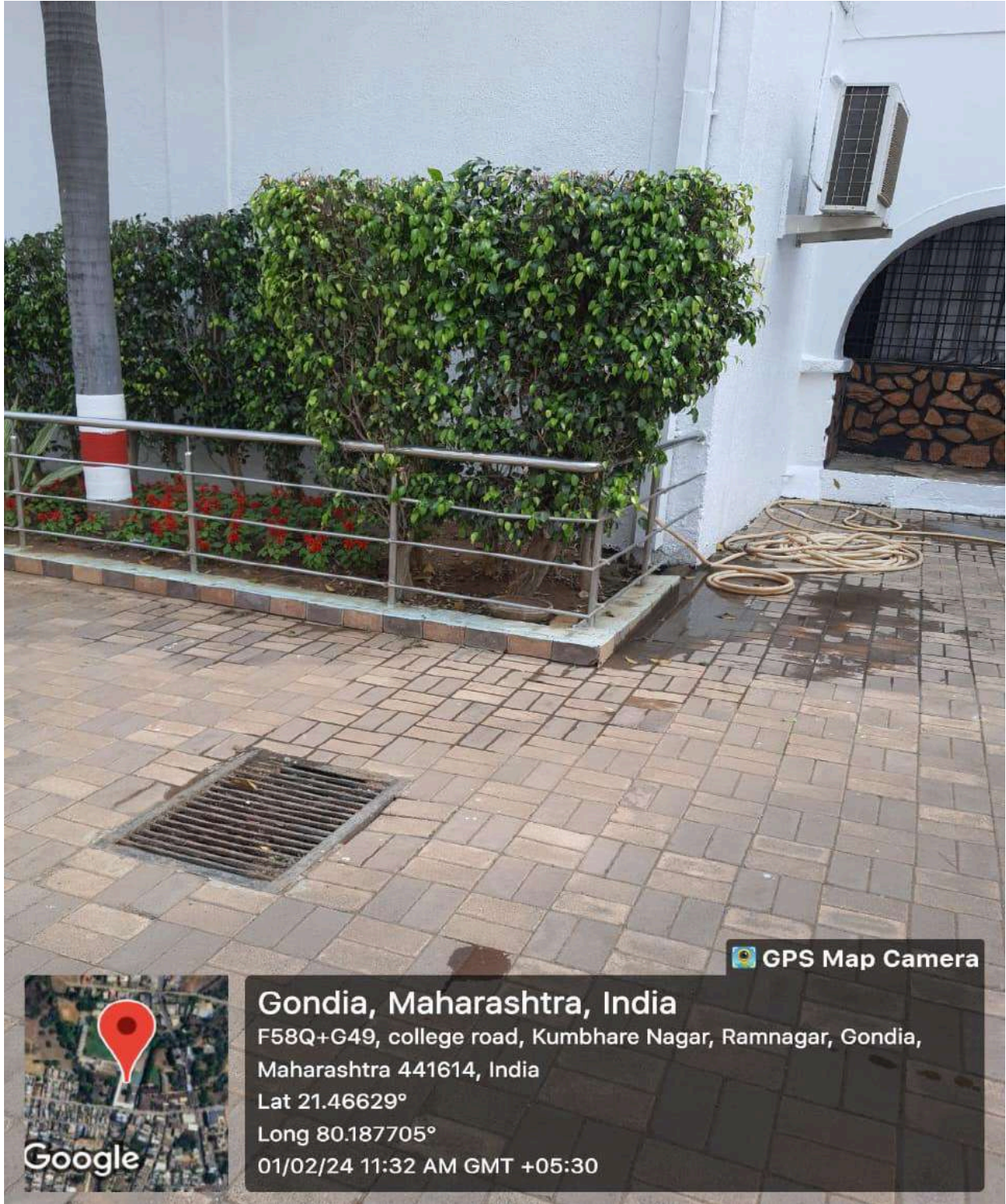
Water Harvesting Chamber
